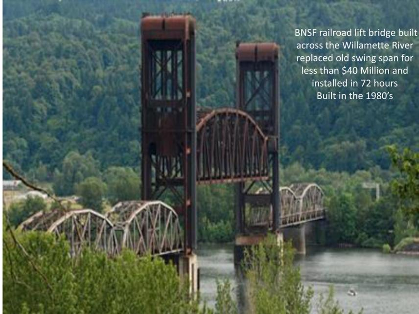
BNSF railroad lift bridge built across the Willamette River replaced old swing span for less than \$40 Million and installed in 72 hours
